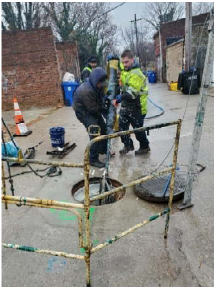
Lateral Lining, CIPP (N Calvert St)
