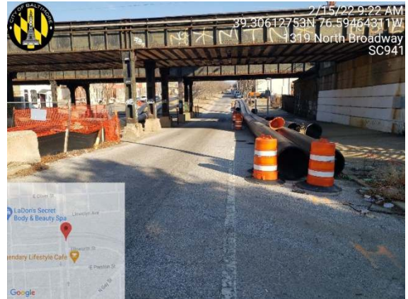
Pressure Sewer (N Broadway)
