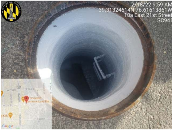
Manhole Rehab (E 21 st St)
