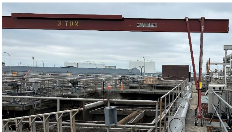
Fig 1: New PST Scum Troughs for Installation
