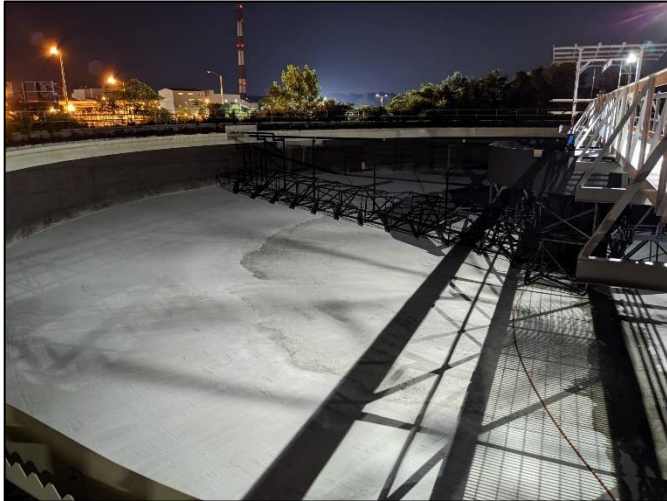
Figure 2: Back River WWTP PST #9 final repairs
