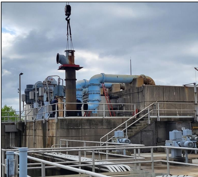
Figure 1: Back River WWTP Outfall 002 Pump Replacement
