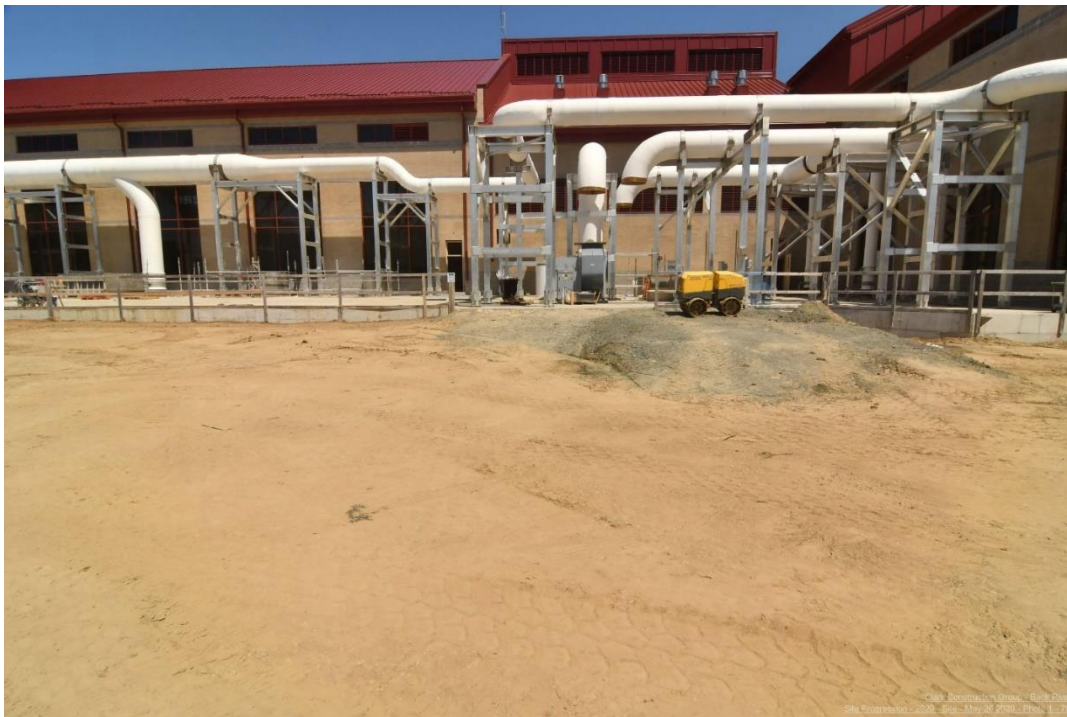
Back River WWTP Headworks Project – IPS Odor Control Ducts; May 2020
