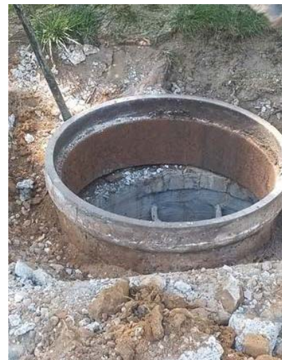
SC 964 adjusting manhole frame and raising to grade
