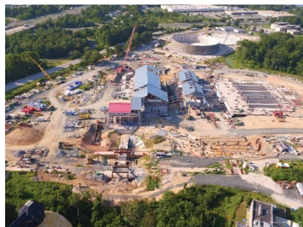
Back River WWTP Headworks Project progress photos June 2019
