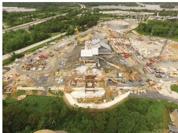
Back River WWTP Headworks Project progress photo April 2019
