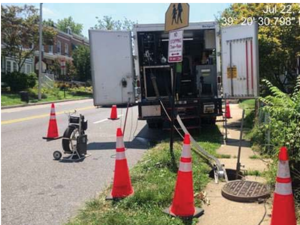
SC 964 non-structural grouting for sewer house connections
