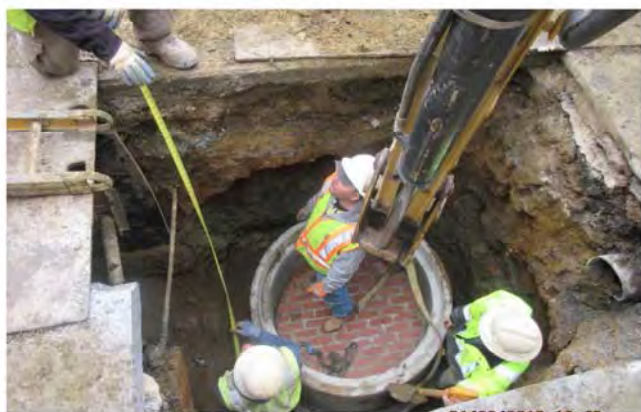
SC 953 new manhole installation
