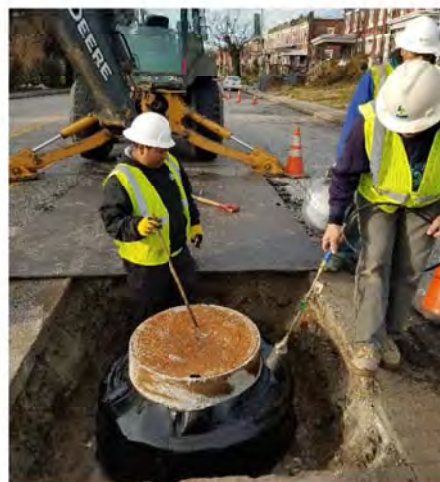
SC 953 installation of external manhole frame seal to curb infiltration
