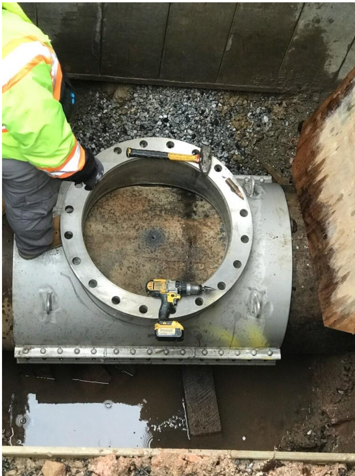
Figure 3-8: SC 941 – Tapping sleeve for bypass
