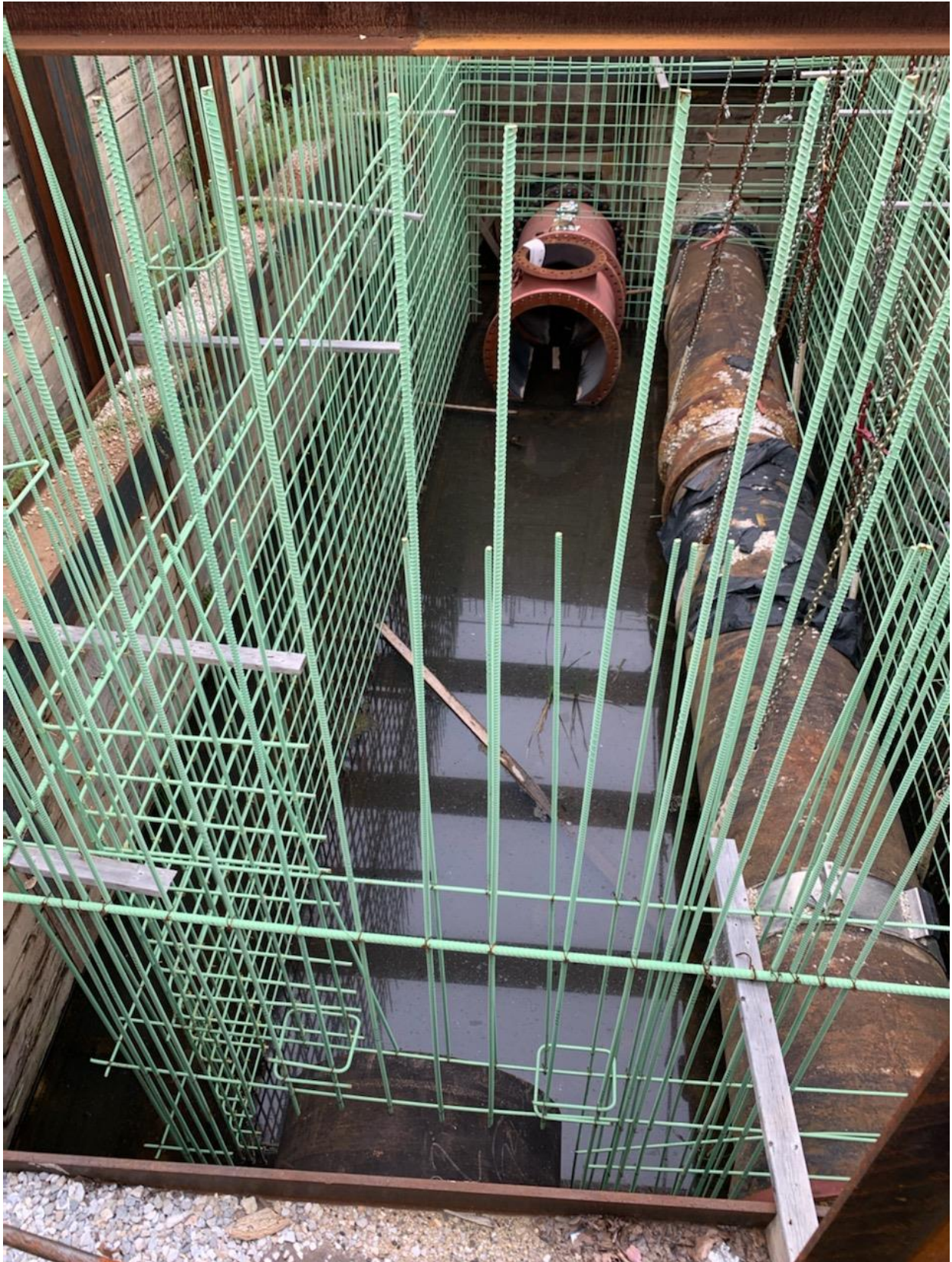
Figure 3-9: SC 941 – Vault 1 rebar
