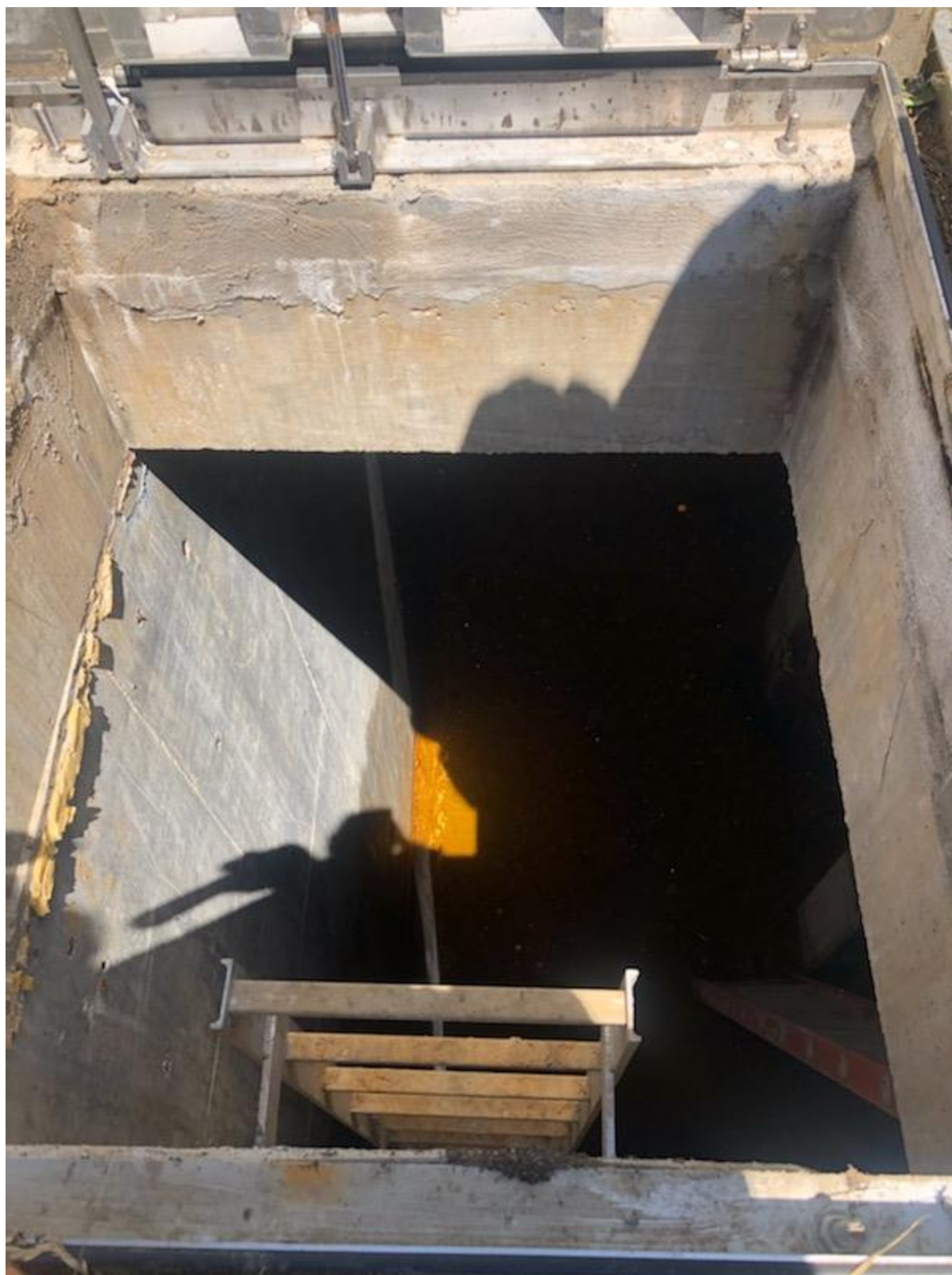
Figure 3-13: SC 963 – Construction of poured-in-place junction chamber
