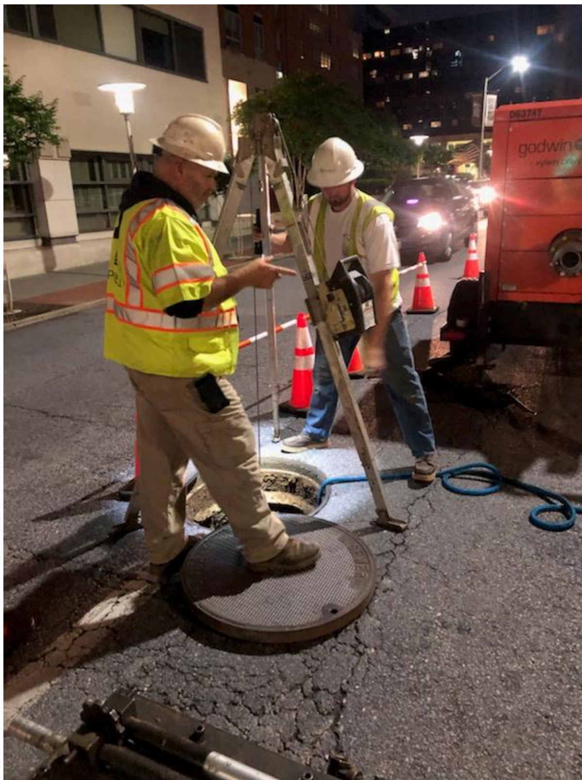
Figure 3-15: SC 963 – CCTV being performed
