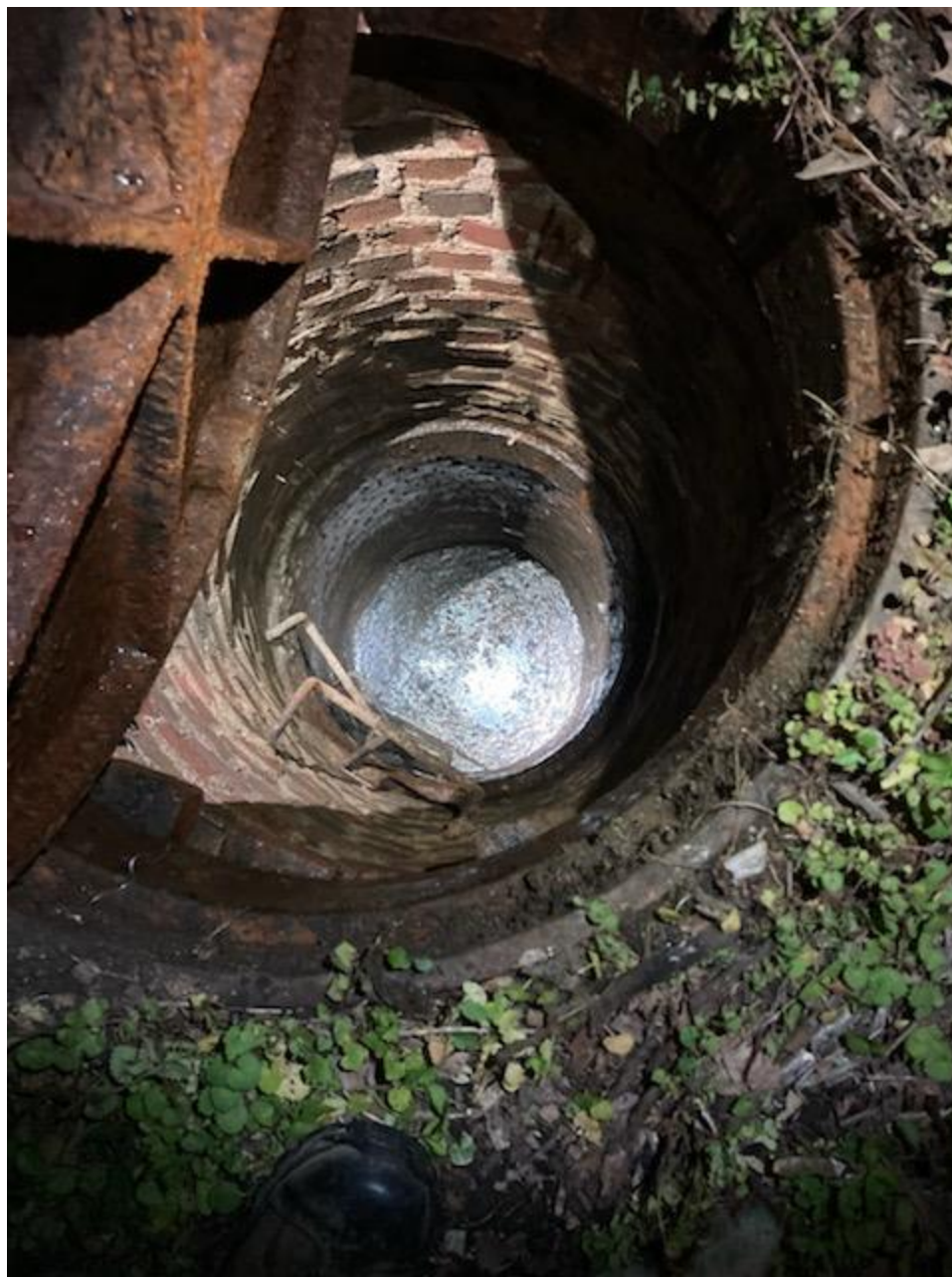
Figure 3-14: SC 963 – Surcharging manhole on 3500 block of Wilkins Avenue
