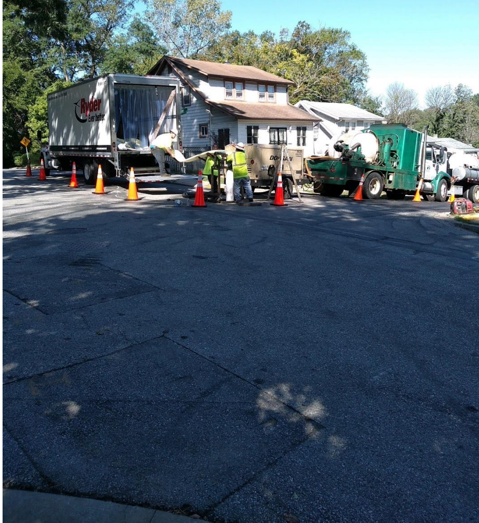
Figure 3-18: SC 977 – CIPP lining
