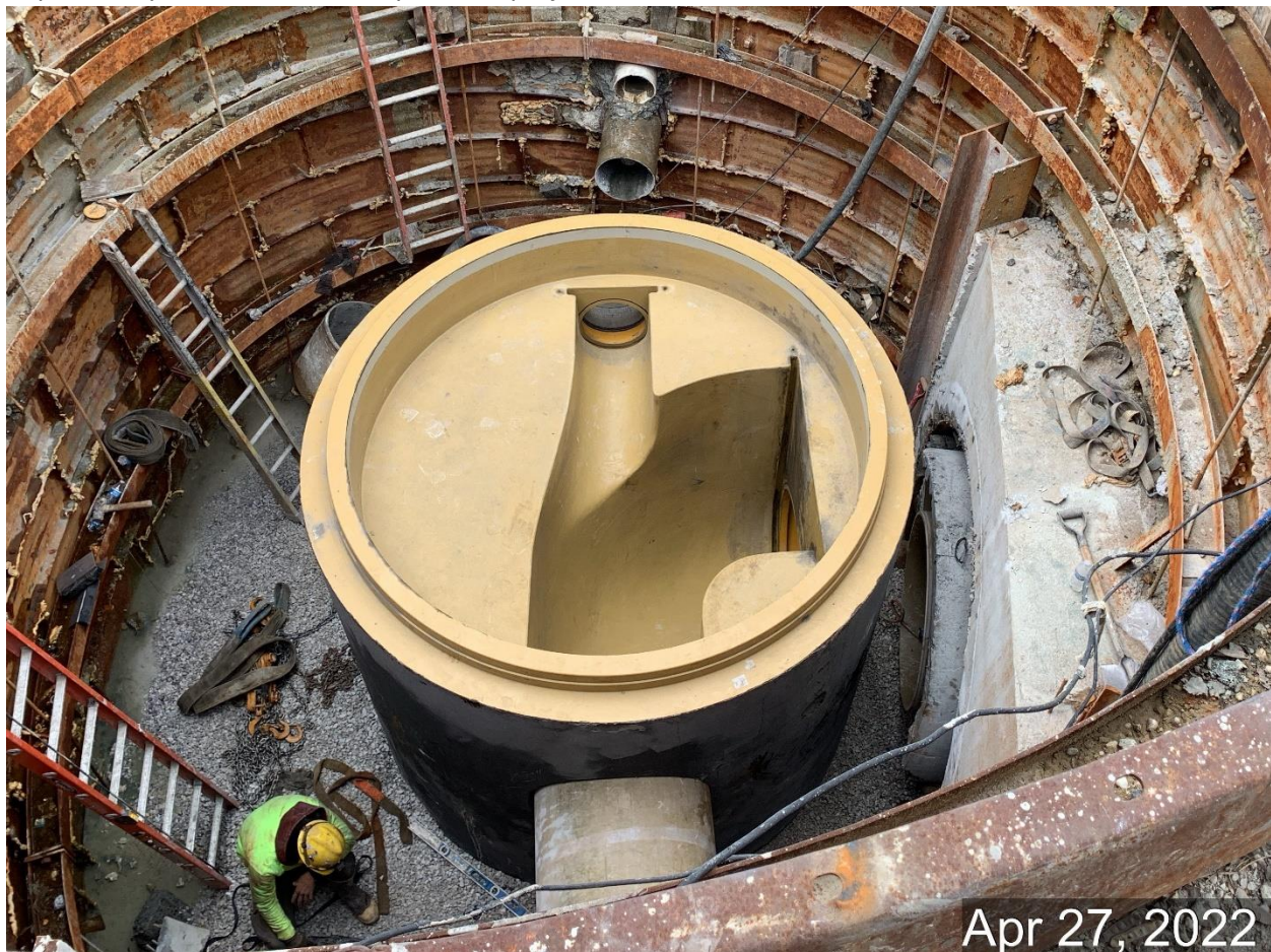
Figure 3-2: SC 940 – Installation of diversion chamber
