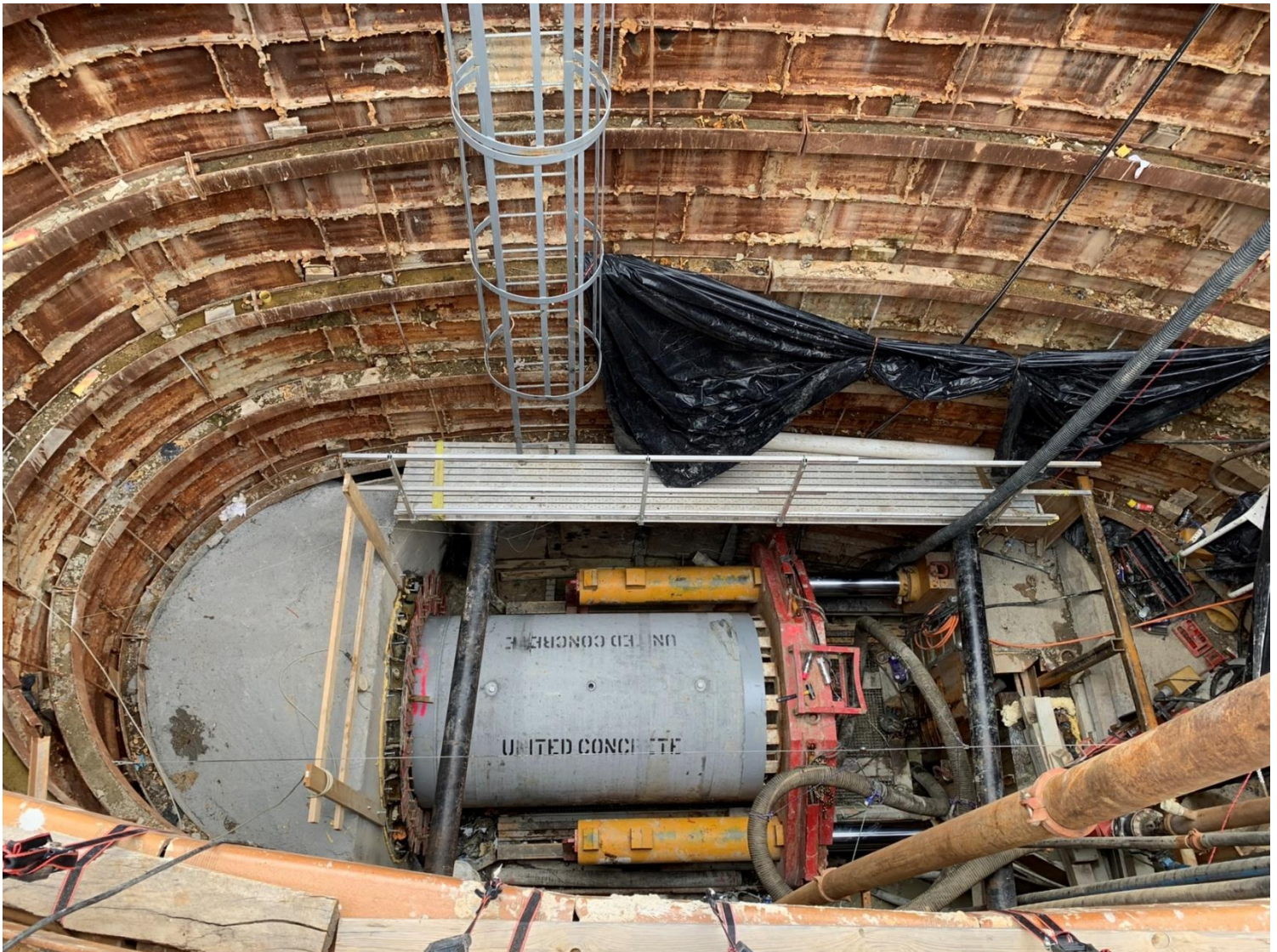
Figure 3-5: SC 940 – Microtunnelling launch pit
