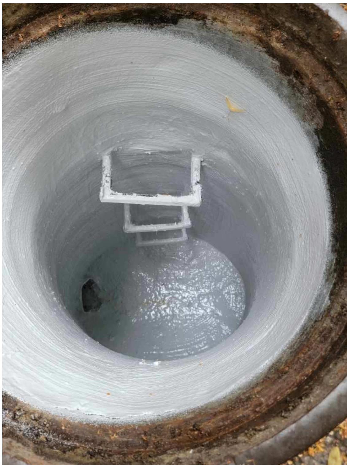
Figure 3-12: SC 941 – Manhole rehabilitation with epoxy coating
