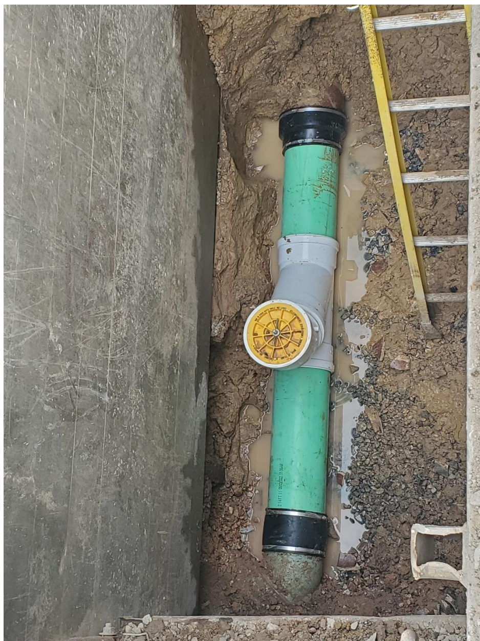
Figure 3-10: SC 941 – Open cut point repair
