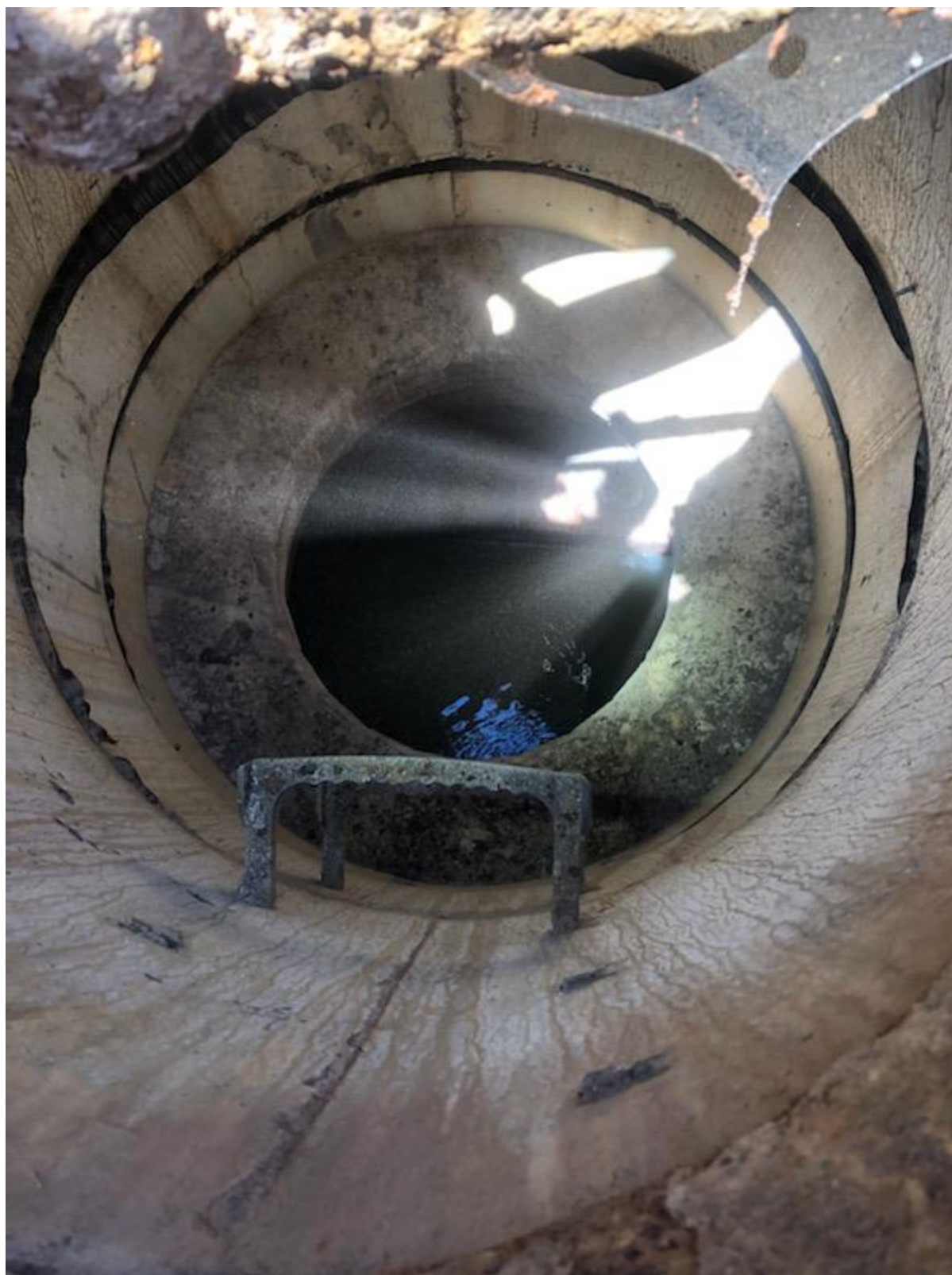
Figure 3-16: SC 963 – Surcharged manhole on 3500 block of Wilkins Avenue
