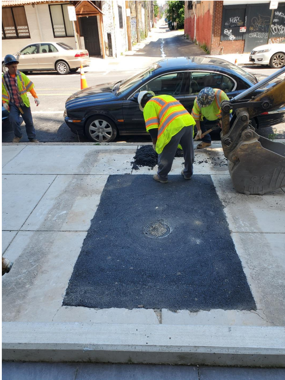
Figure 3-8: SC 941 – Temporary sidewalk asphalt patch
