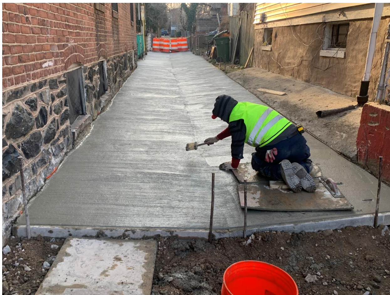
Figure 3-19: SC 977 – Concrete finishing and site restoration in alley
