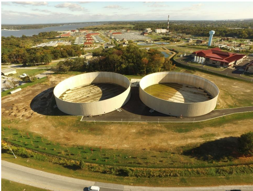
Back River WWTP Headworks Project – EQ Tanks ; December 2021
