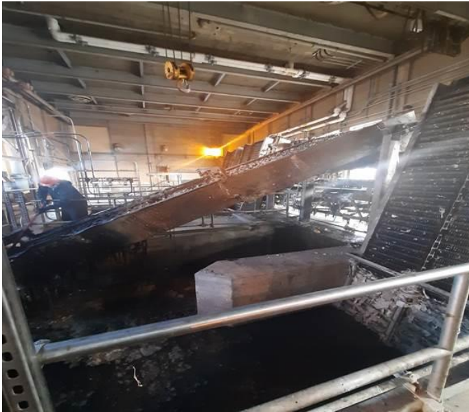
1 Removal of fine screens for refurbishment
