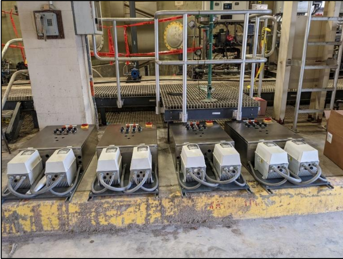
Figure 2: Back River WWTP new polymer units ready for installation
