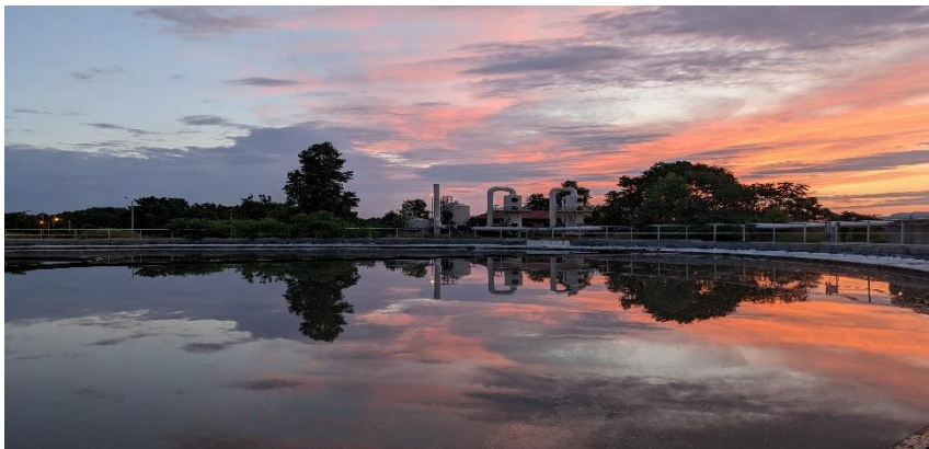
Figure 1: Back River WWTP Primary Settling Tank
