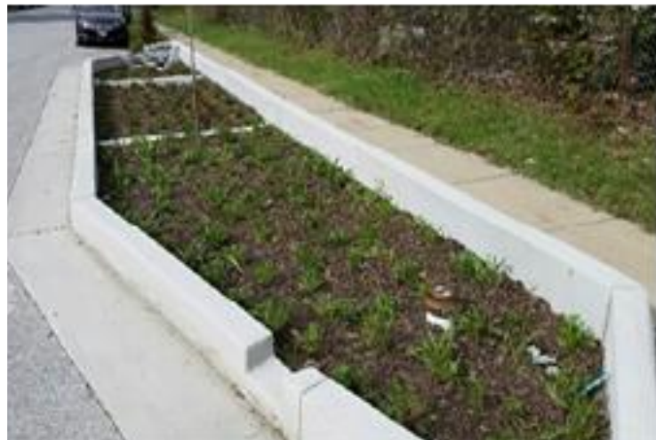
Stormwater Bumpout facility at Bush Street
