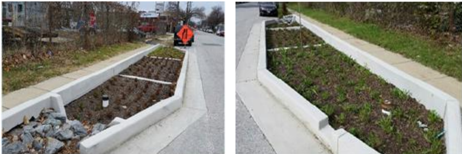
Stormwater Bumpout facility at Bush Street
