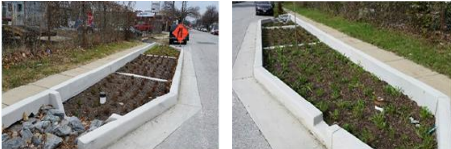
Stormwater Bumpout facility at Bush Street
