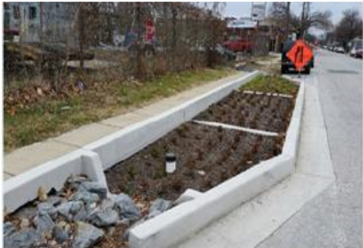
Stormwater Bumpout facility at Bush Street
