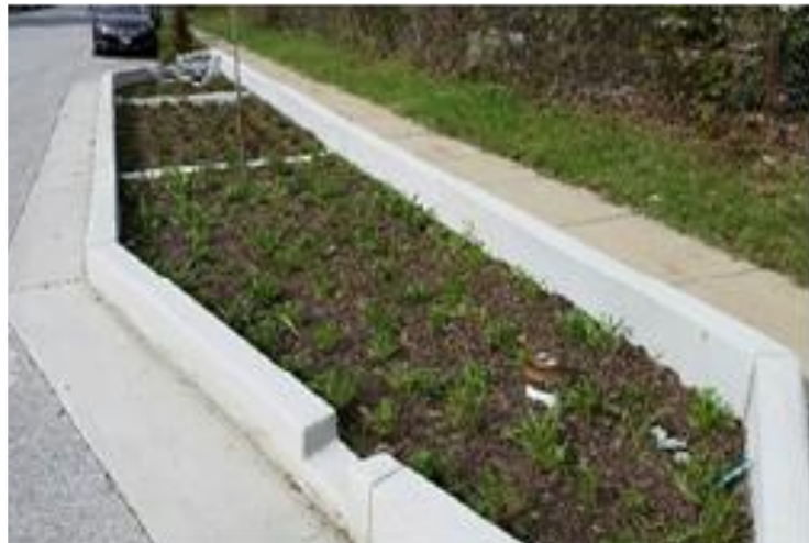
Stormwater Bumpout facility at Bush Street
