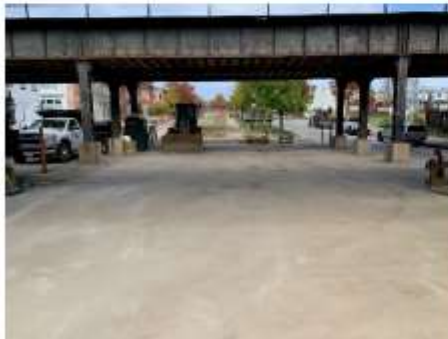
SITE CLEANED UP
