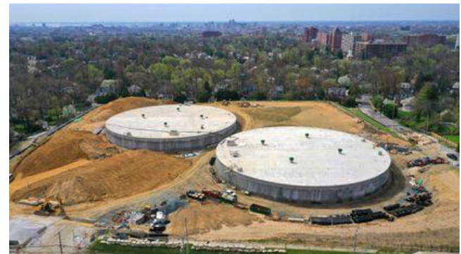
Guilford Reservoir covered tanks construction underway.
