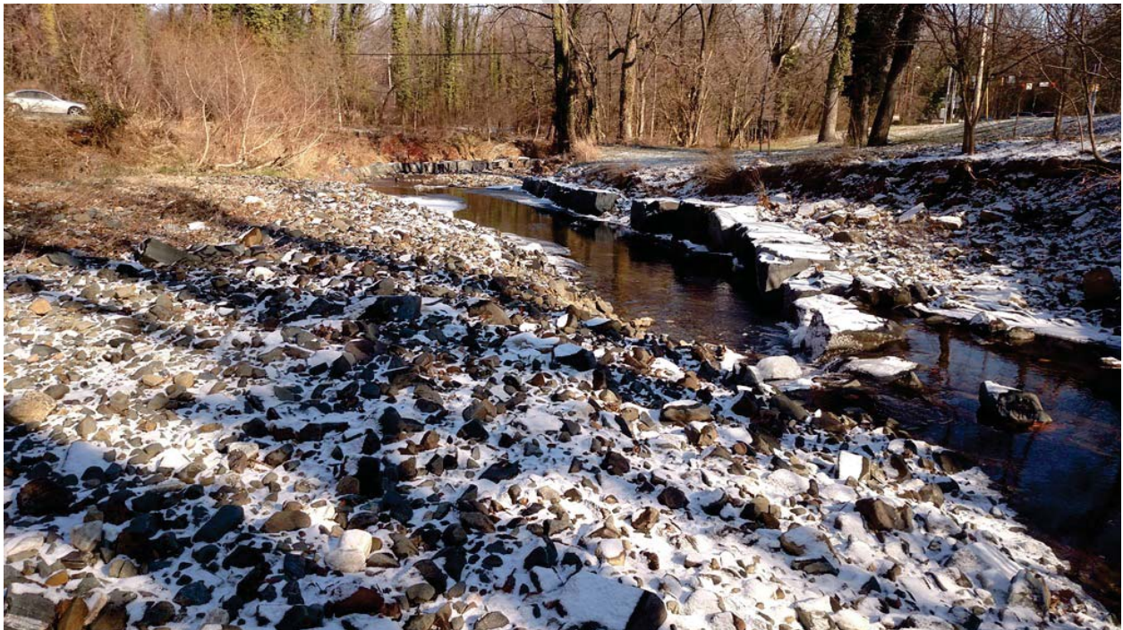
Photo 24. Western Run. Excessive deposition covering cross vane 2.
