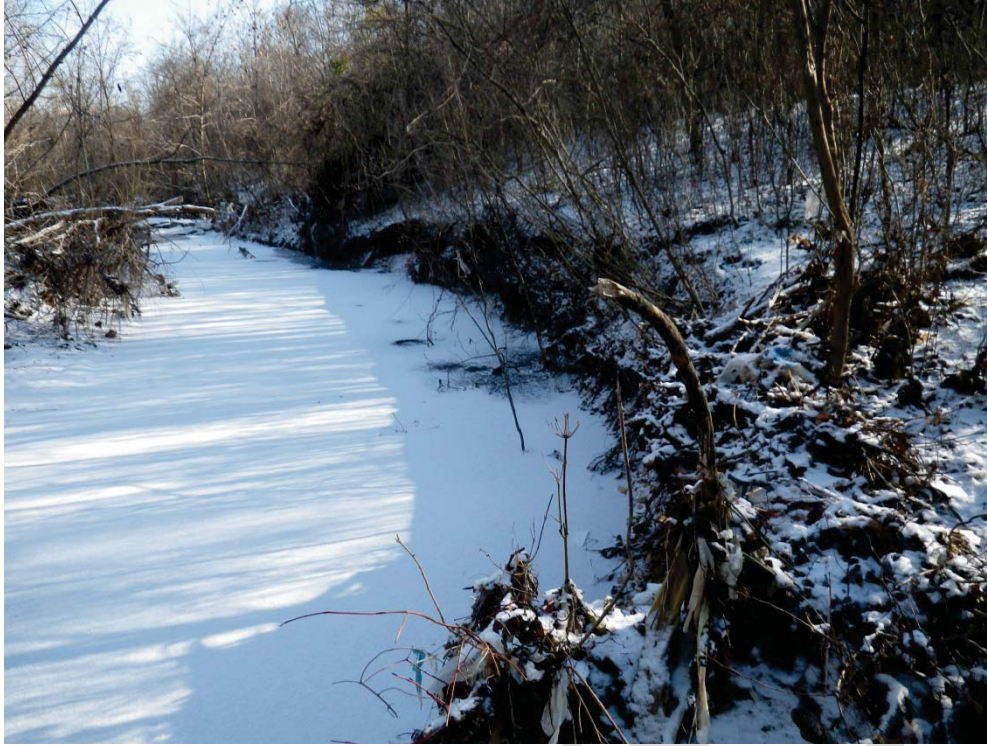
Photo 15. Biddison Run. Major bank erosion on right bank of station 07+70 – 08+35.
