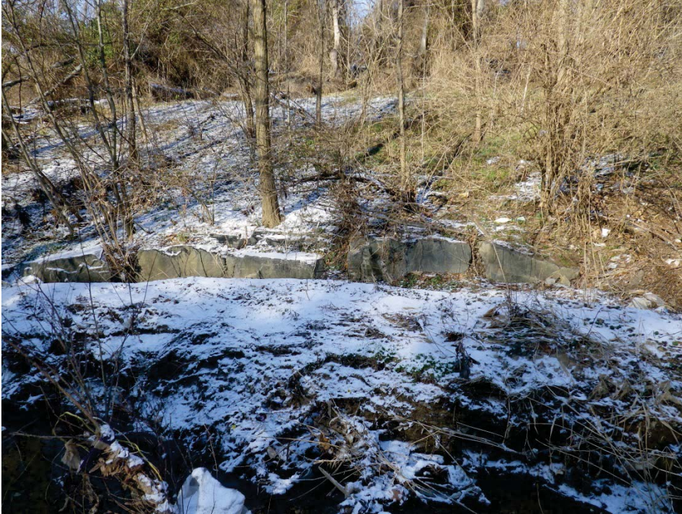
Photo 13. Biddison Run. Excessive sediment deposition in front of imbricated wall station 01+60.
