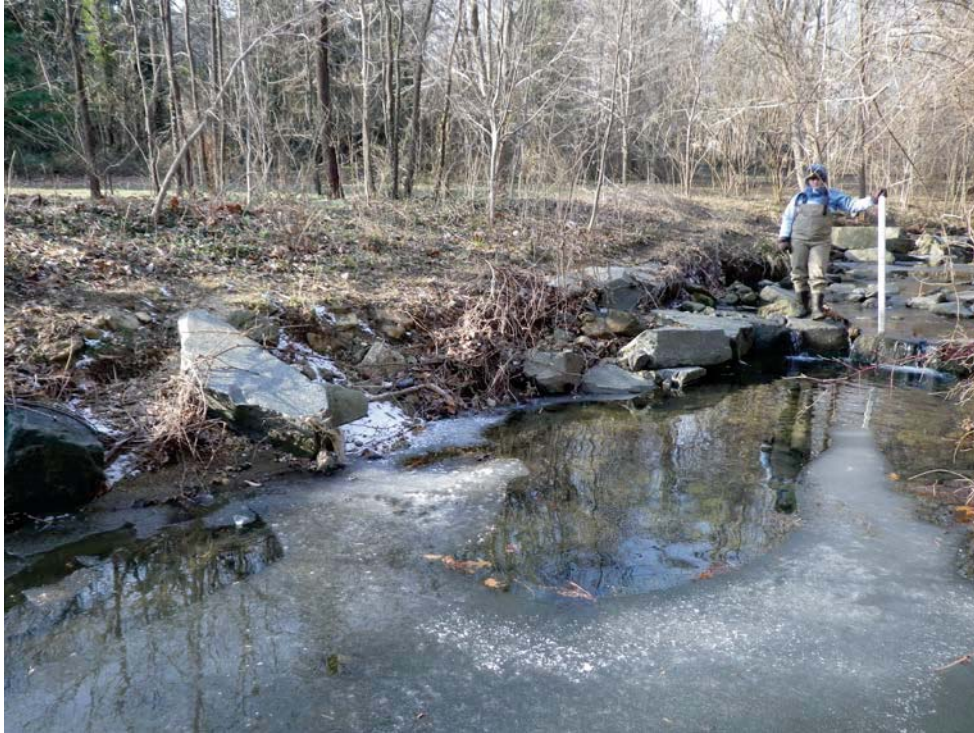
Photo 11. Middle Stony Run. Right bank erosion causing failure of cross vane 8 right vane arm at station 14+61.
