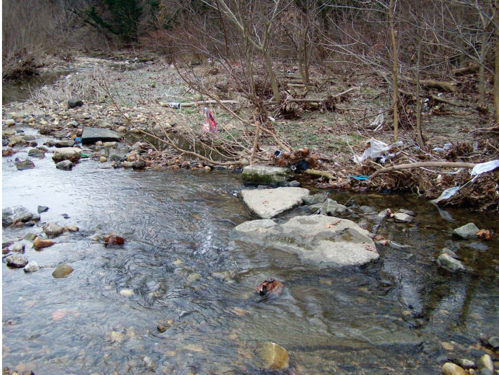
Photo 20. Maidens Choice. Station 06+00. Stream structure right arm buried from sediment.
