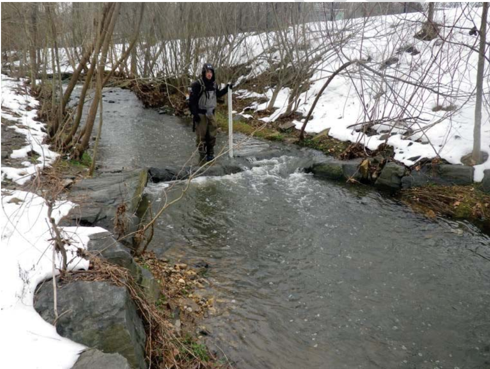
Photo 3. Upper Stony Run. Cross vane at station 25+95 showing typical structure issues and results: scour on upstream of vane arm and deposition along downstream vane arms.
