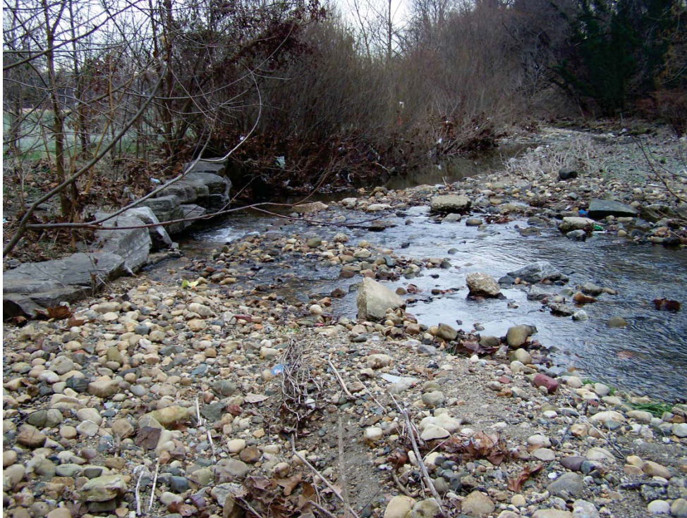
Photo 19. Maidens Choice. Station 06+00. Stream structure with pool filled in with sediment.
