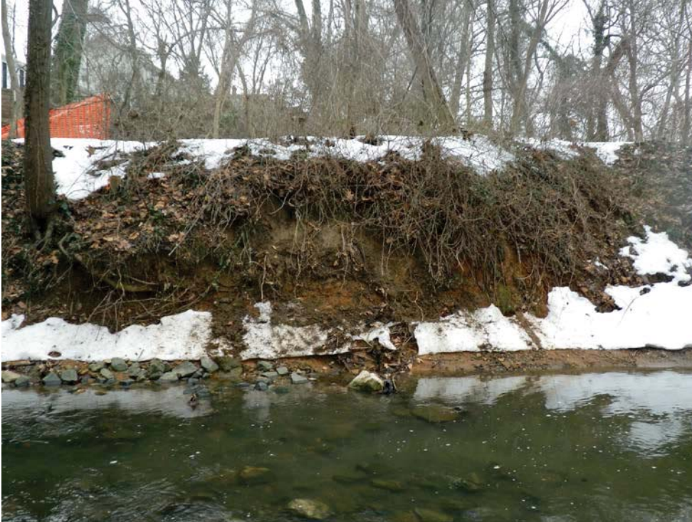
Photo 6. Upper Stony Run. Right bank erosion at station 27+40.
