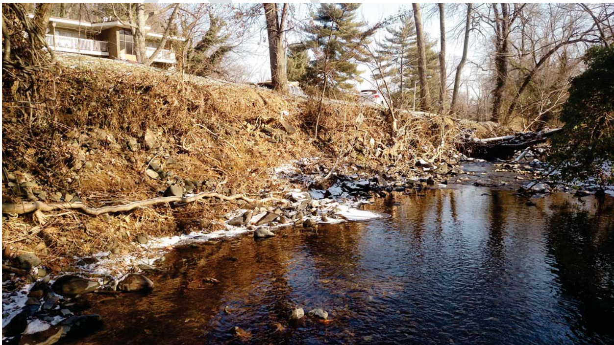
Photo 22. Western Run. Lateral bank erosion.
