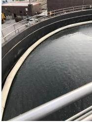
Repairs to the Gravity Sludge Thickener (GST) #4, pictured left, have been completed and returned to service. This repair provides all three operational GSTs for Patapsco Waster Water Treatment Plant (PWWTP). The optimal number for average plant flows is two GSTs.
