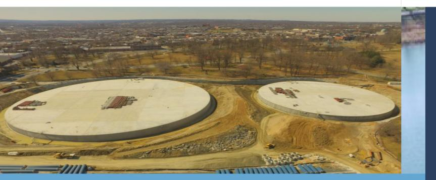
The City's iconic Druid Lake holds filtered and treated water that is ready to be delivered to consumers. At this site, two massive underground tanks are being built to protect this drinking water supply.
