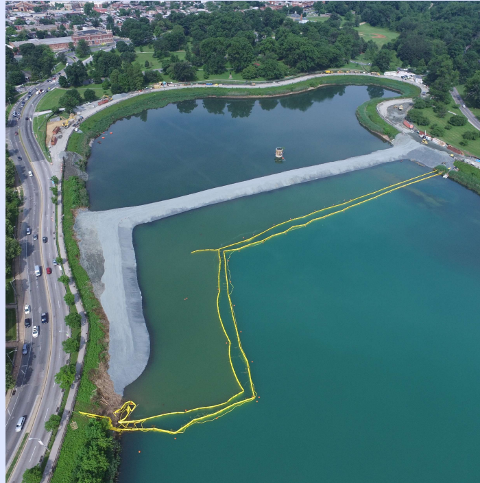
Cofferdam & Turbidity Curtain Completed - 6/8/2018
