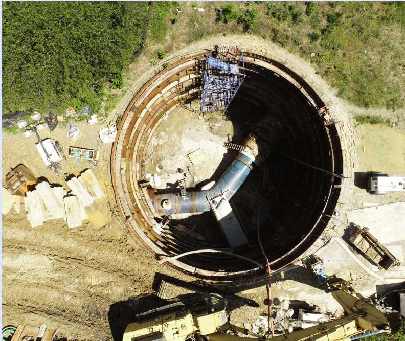
Alignment A – Tie-in Piping – 5/13/2024
