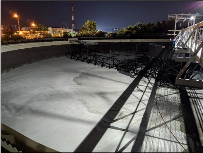
Figure 2: Back River WWTP PST #9 final repairs
