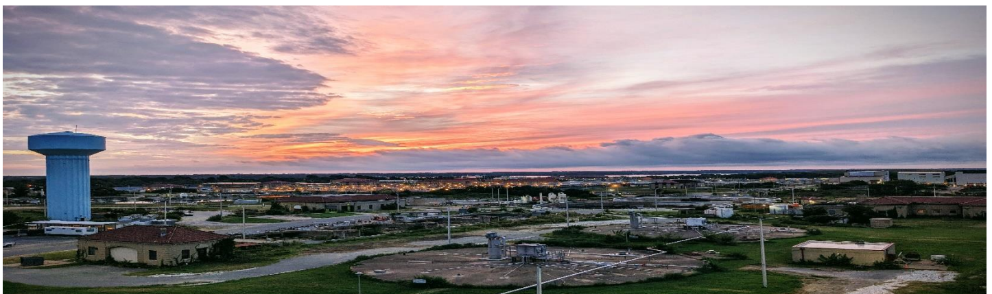
Figure 1: Aerial View of Back River WWTP
