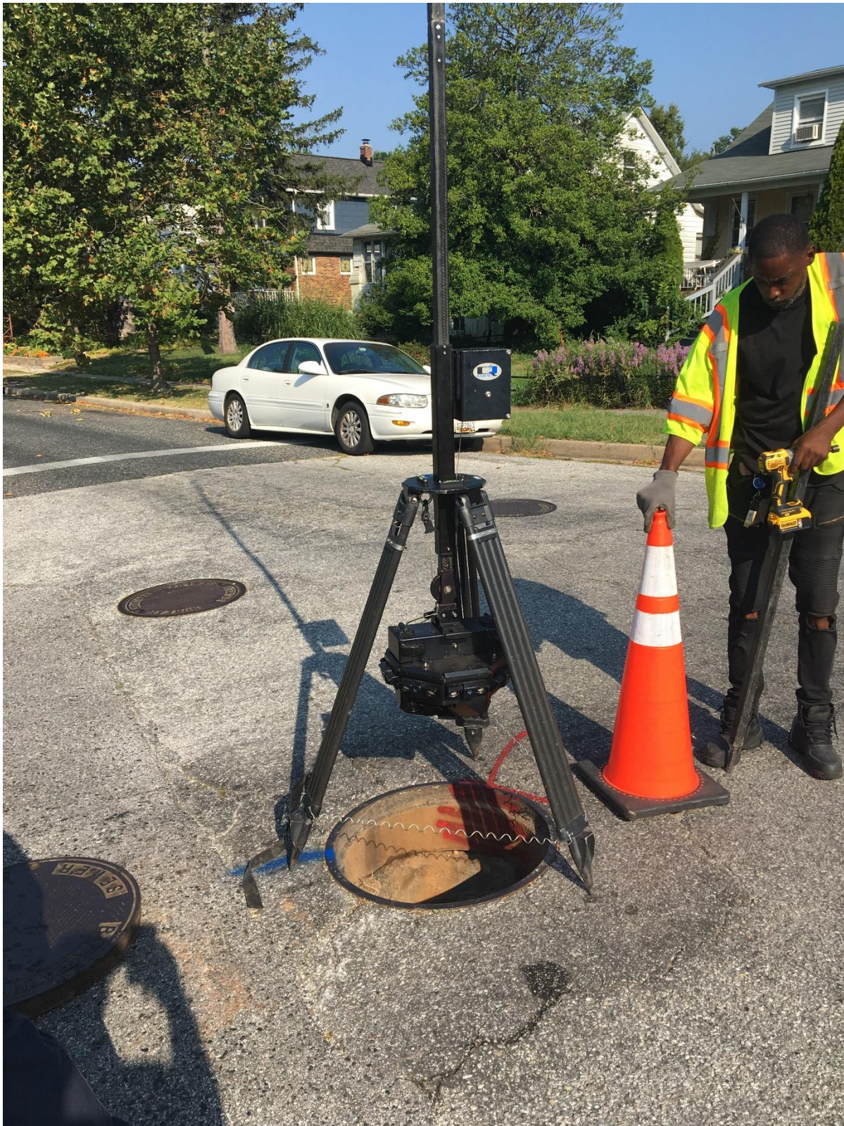
Figure 4-3: SC 1019R – Beechland Avenue - Manhole inspection
