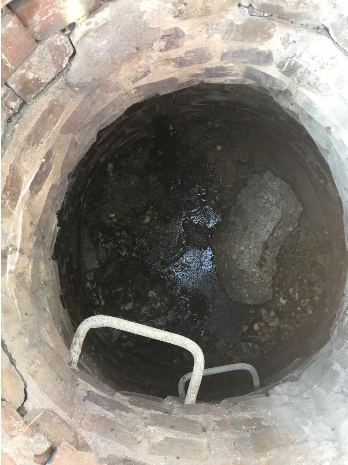
Figure 4-2: SC 1019R – Tramore Road - Manhole inspection
