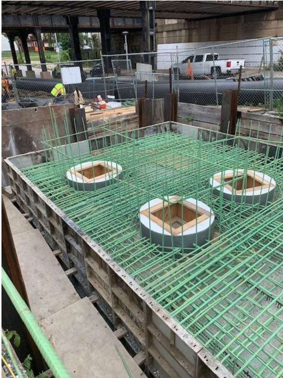
Figure 3-5: SC 941 – Vault 1 rebar installation
