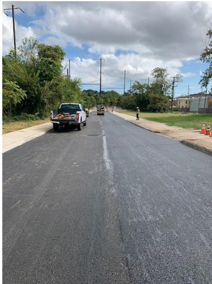
Figure 3-2: SC 941 – Asphalt completion of 1700 Ellsworth Street
