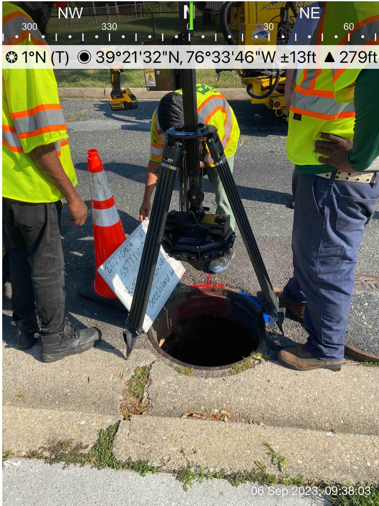
Figure 4-4: SC 1019R – Beechland Avenue - Manhole inspection
