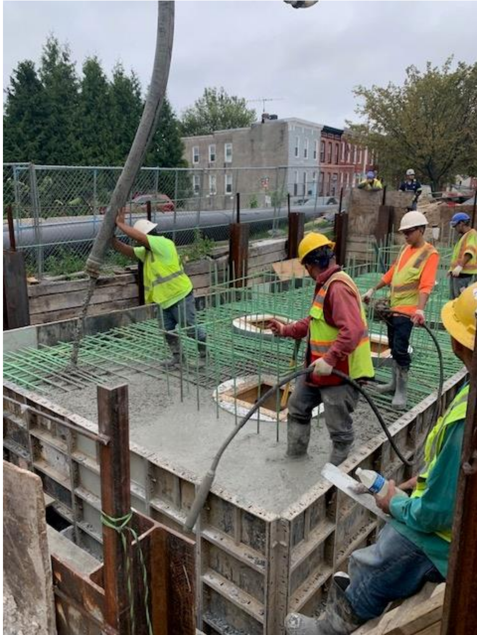
Figure 3-4: SC 941 – Vault 1 concrete pour for top slab
