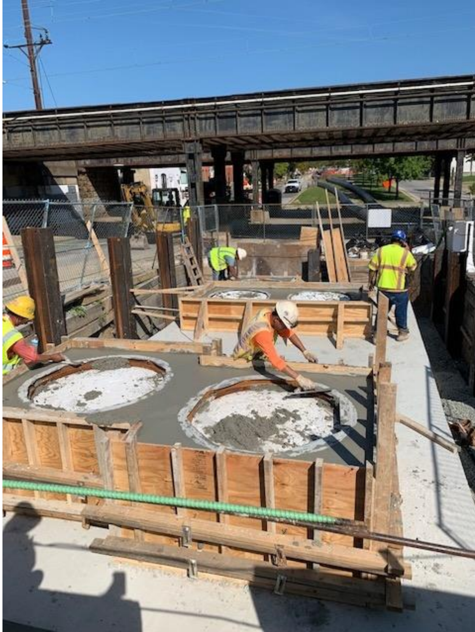
Figure 3-3: SC 941 – Vault 1 concrete pour for Manhole risers
