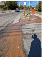
2. Please install inlet protection and pump into filter bags. Each hose should have its own filter bag.
