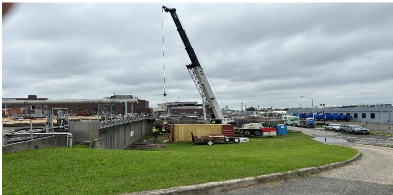
Fig 1: PST Scum Trough Repairs
