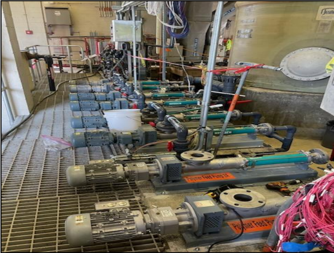
Figure 2 New Polymer units installation nearing completion
